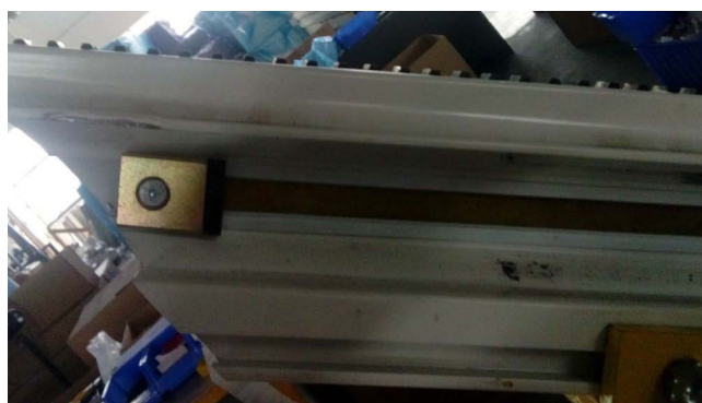
Figure 32: Bus line stopper installed on rail
