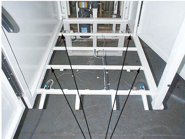
Figure 33 Install cab floor panel
